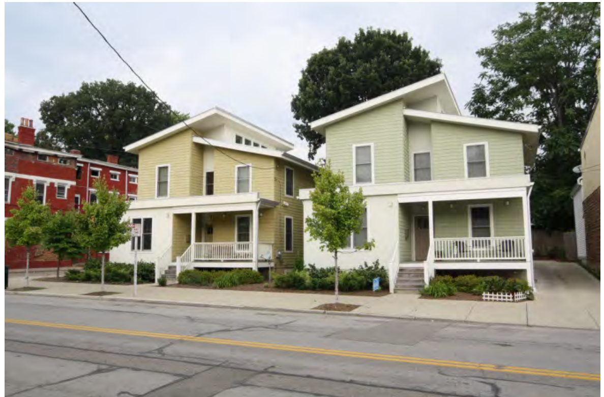
CNCURC recently completed these two homes on Chase and Fergus
