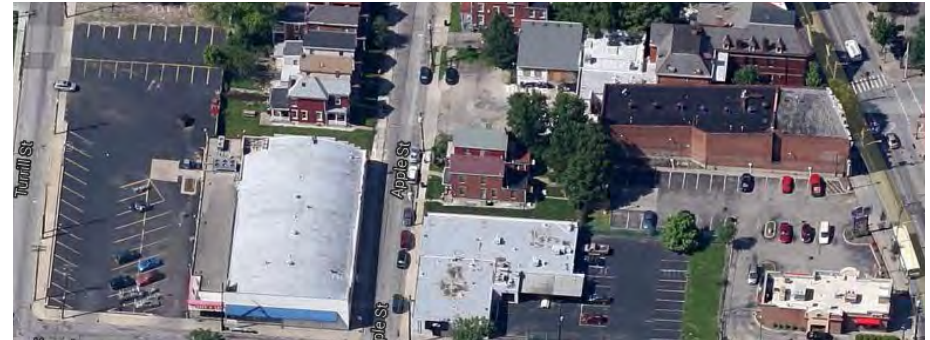
The Save-a-Lot site is at the far left, with the business district on the far right
